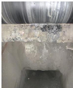
Gambar.1 Built-up material di chute inlet mill
