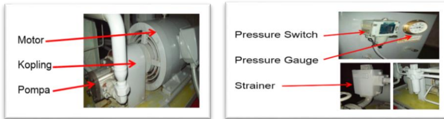
Gambar 2.1 bagian-bagian pompa Oil Lifter
