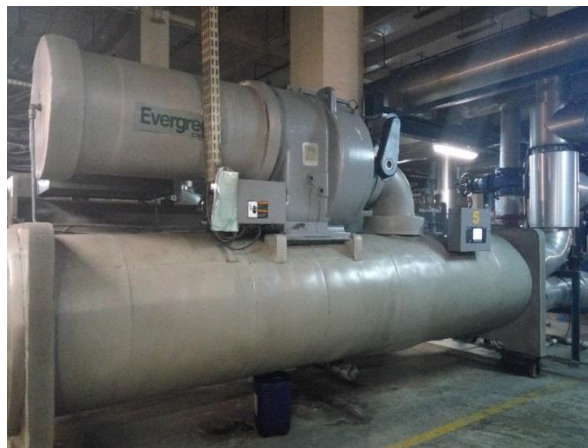
Gambar 1.1 Chiller water cooled
