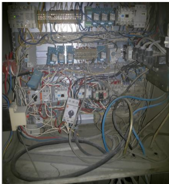
Gambar.2 Sistem Kontrol 622 BB1 Sebelum Upgrade
